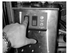
1. Energize boiler and fill to operating level.
